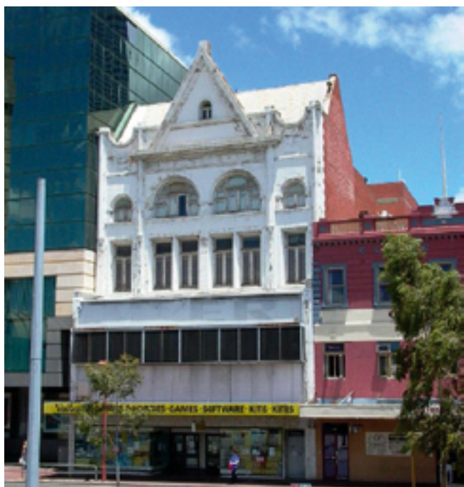
ABOVE: Baird's Building (fmr), Perth - before removal of paint
